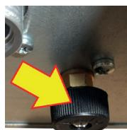
Restore the correct pressure value by acting on the boiler filling valve (for optimum operation, the pressure value should be within 0.8 and 1 bar).
